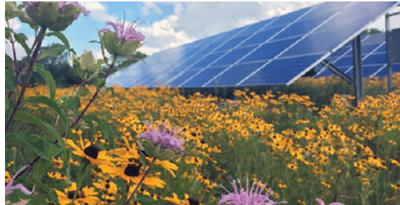
Westmoreland Schools Solar Habitat (from the web)
